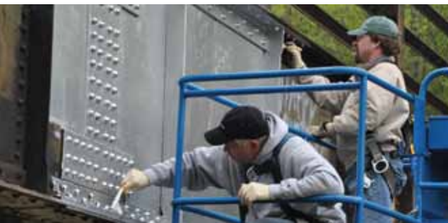
POET Biorefining – Hanlontown team members sprucing up the bridge.
